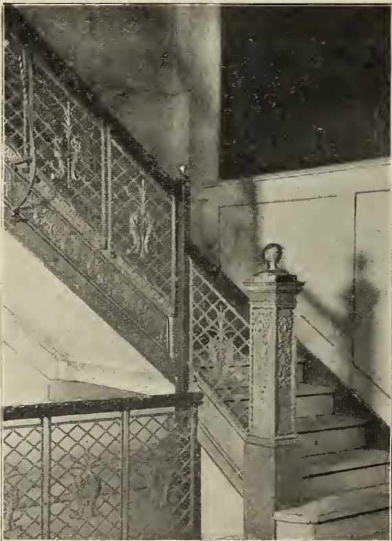
C.—STAIRWAY, VENETIAN BUILDING, CHICAGO. Aluminium.
